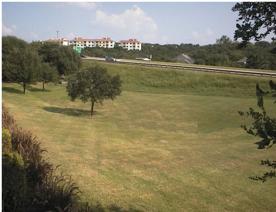
Figure 4-29 Example of an Infiltration Basin
