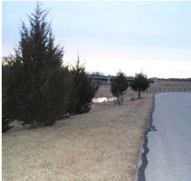
Figure 4-17 Filter Strip
